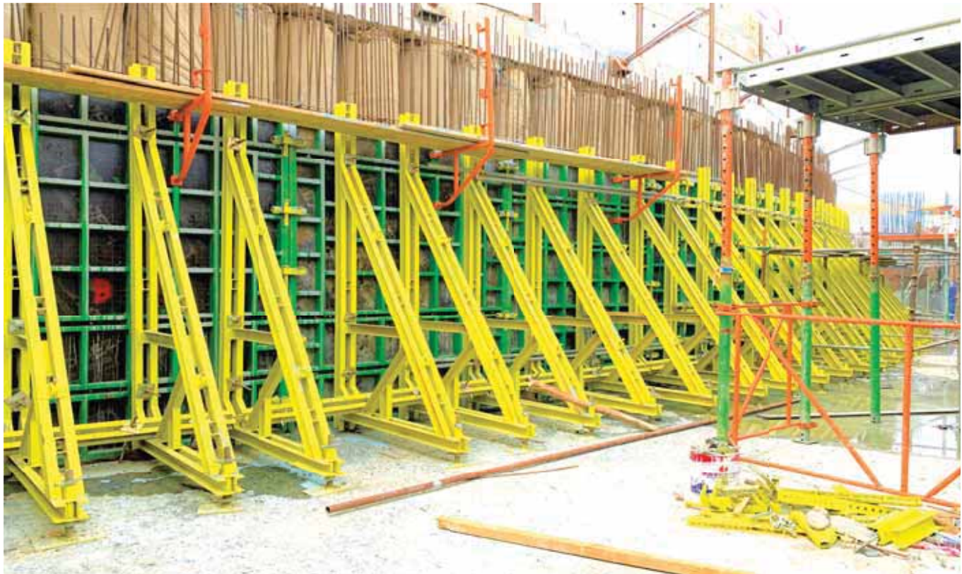
TB1 Retaining Wall
