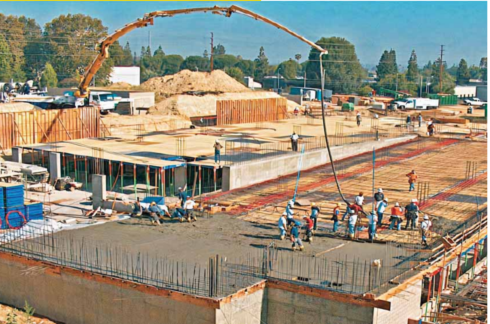
Concrete being pumped onto typical ramp constructed using TABLA Shoring.
