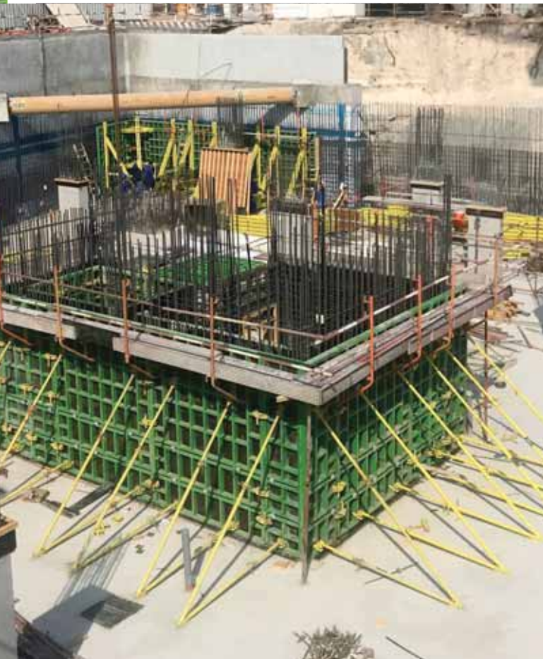
The frame and panel are the heart of the new TABLA Wall Form System.
