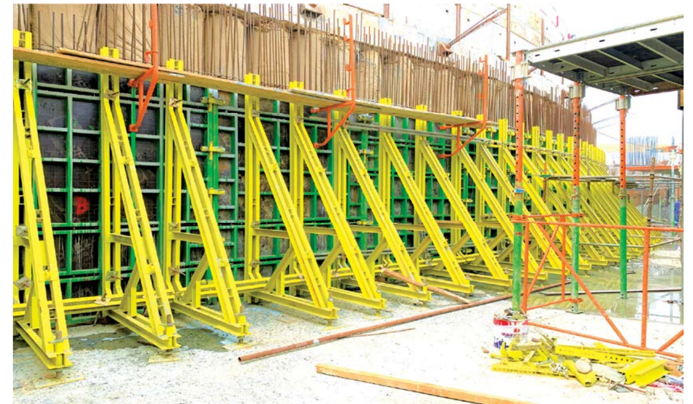
TB1 Retaining Wall
